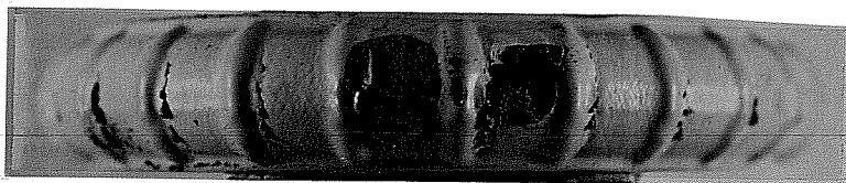
Figure 6.6 Deterioration of Exposed Areas on 13-mm Bar with Parallel Deformations.
