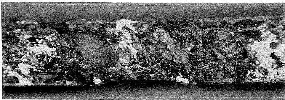
Figure 11.26 Corrosion of Uncoated Compression Bars at Crack Location.
