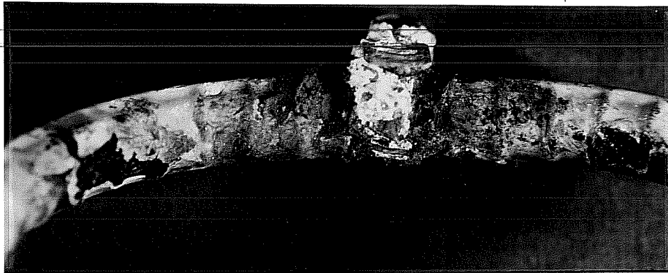
Figure 11.21 Corrosion at Areas of Contact Between Patched Stirrup and Uncoated Bars.
