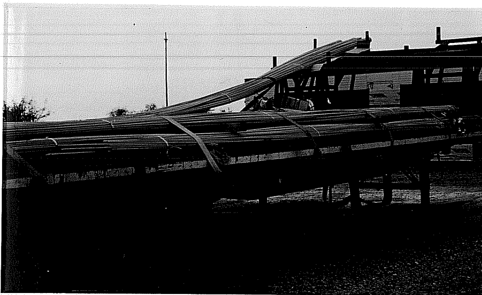
Figure 3.16 Transportation of Epoxy-Coated Reinforcement.
