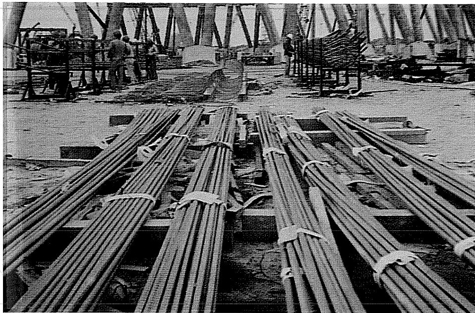
Figure 3.18 Proper Storage of Coated Reinforcement. 84
