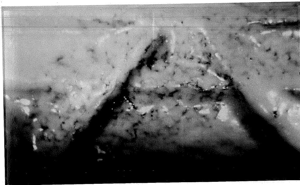
Figure 3.9 Improperly-Coated Reinforcing Bar Surface Near the End.
