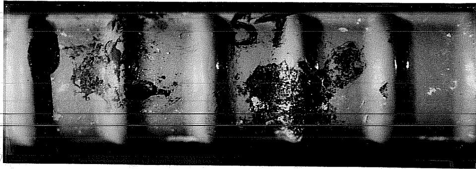
(a) Damaged Upper Bar from Cracked Unloaded Beam B9
