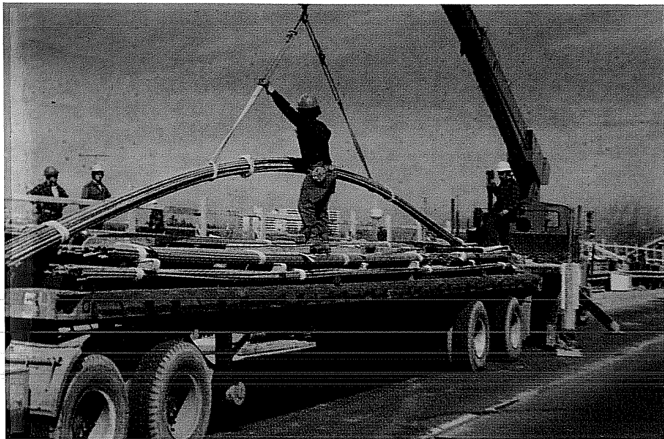
Figure 3.15 Hoisting of Coated Bars with Multiple Lift Points. 86
