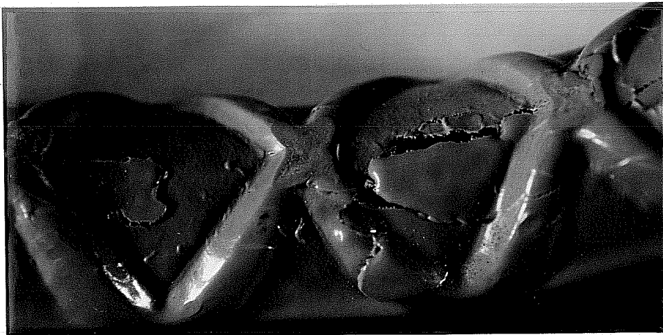
Figure 3.12 Damage on the Inside Surface of Bent Bar.
