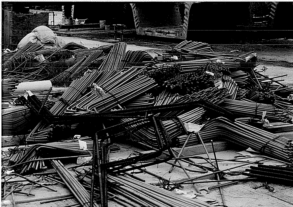
(b) Inadequate Storage of Coated Bars at the Job Site
